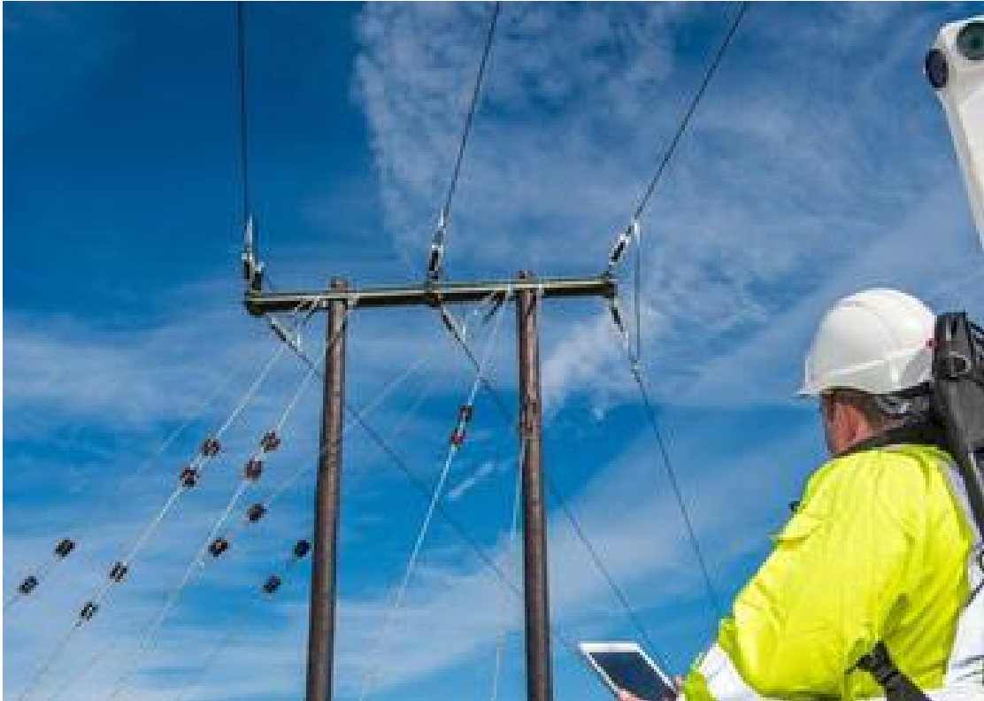
FIGURE 2.2: Foot patrols as means of inspection.
