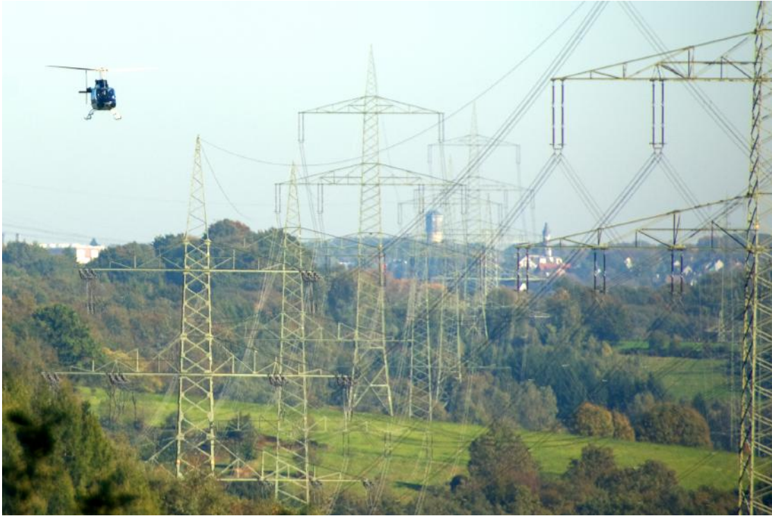
FIGURE 2.3: Helicopter used for power line inspection.
